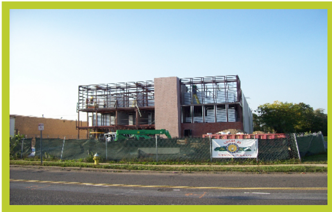
Deer Park Storage on Long Island, NY – under construction.
