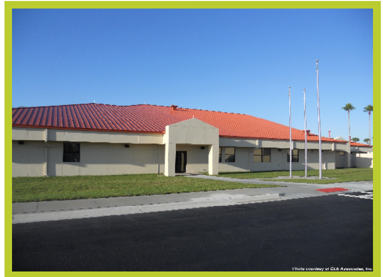
MacDill AFB Building 53 Roof Retrofit project, Tampa, FL.
