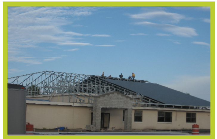
MacDill AFB Building 53 Roof Retrofit – under construction.
